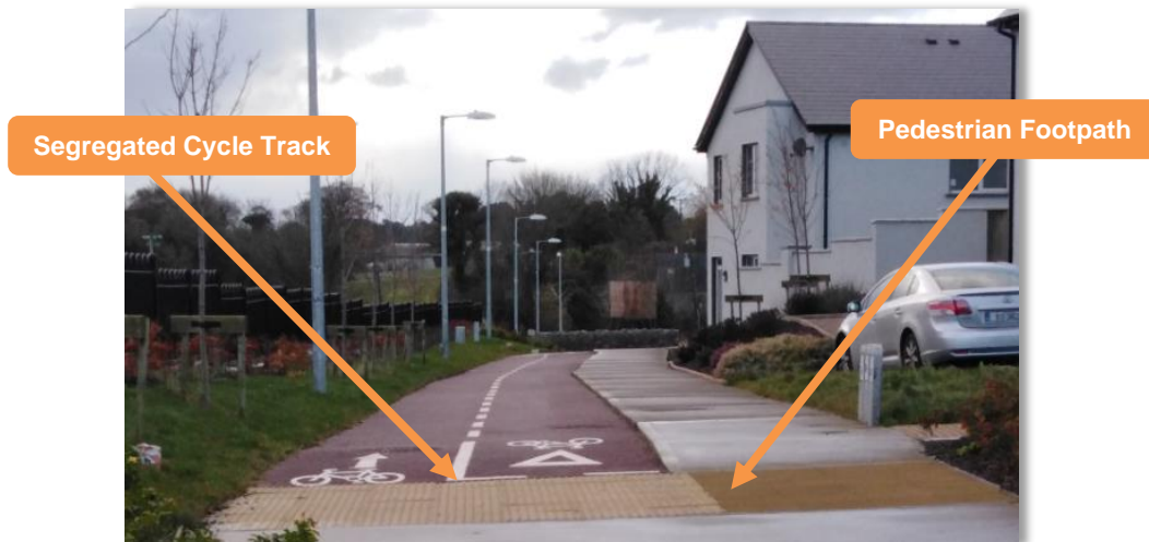
Photo 2: Pedestrian and Cycling Facilities At Ballygossan Park (Cabra Hill Entrance)
