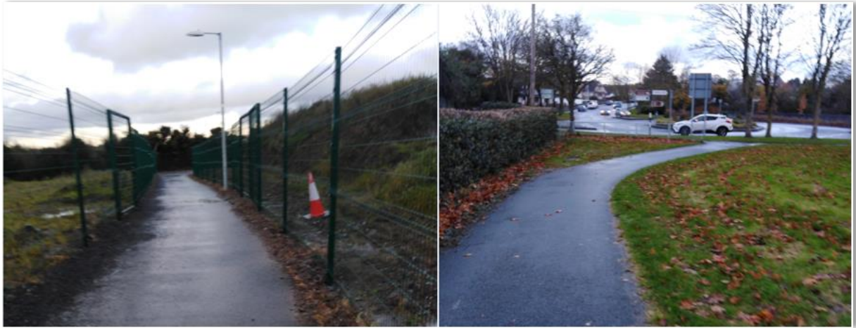
Photo 1: Existing Pedestrian / Cycle Connection between Ballygossan Park and R127 Skerries Rd
